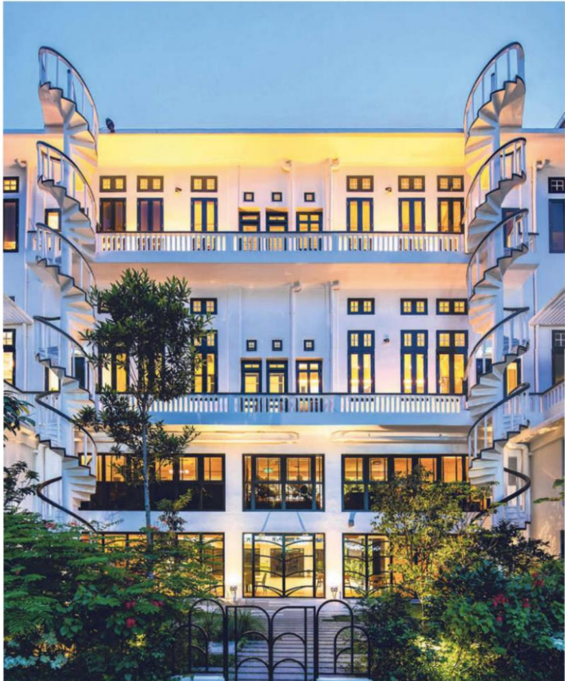
The conservation of Temasek Shophouse in Orchard Road started in 2018 and took 18 months to complete. PHOTO: SURBANA JURONG
